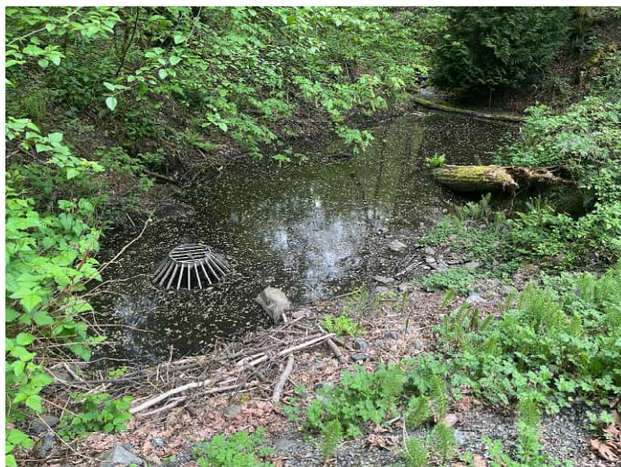
A view of the sediment pond at E Mercer Way, facing upstream.
